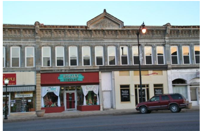
The Summit Block at 316-318 S. Summit is an excellent example of an Italianate facade with ornate cornice, arched windows and cast-iron columns.
