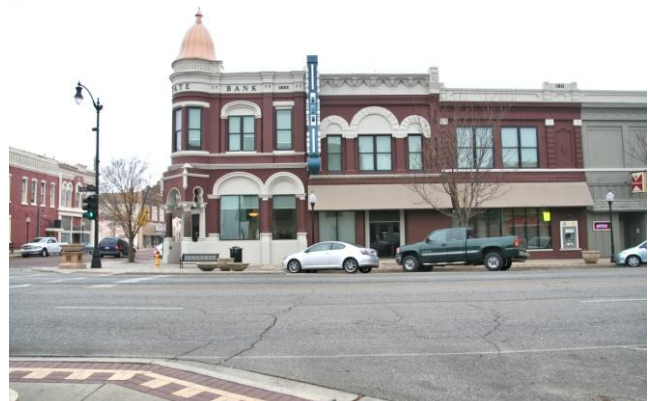
The Union State Bank Building at 127 S. Summit is an excellent Late Victorian example with the heavy arched stone lintels reflecting Richardsonian Romanesque influences.
