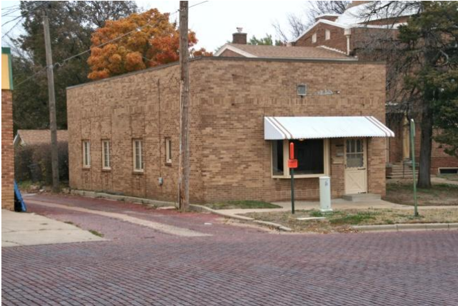
The Christian Science Reading Room Building on E. Chestnut reflects the Minimal Commercial style in a simple commercial building with punched window and door openings. Original steel casement windows remain intact on the east and west sides of the building.
