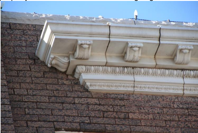
Glazed terracotta cornice on the old Barnard's Ladies Wear Building on S Summit.
