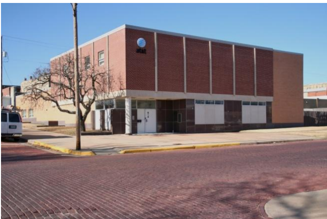
Built for Southwestern Bell in 1960, the building located at the corner of E. Adams and S. A Street reflects Post-WWII Modern styling with an asymmetrical facade composition and varied materials and textures to provide articulation of the facade.
