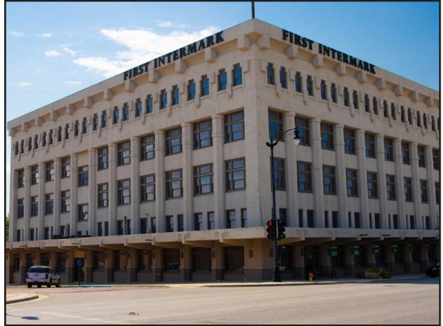
and Adams Avenue, defined by its plentiful windows and geometric trim elements. The stucco-covered building occupies a space of 100 by 132 feet and is solidly built of reinforced concrete, with recessed windows that provide plenty of light. Entrances to the building are on Adams Avenue and Summit Street.
